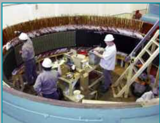
On-site hydro generator rewinds
