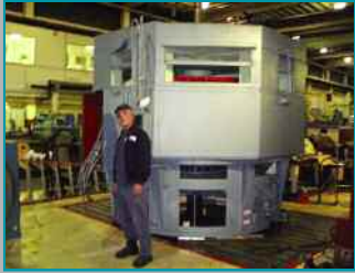
Testing to 750 kVA – 4,160 V, 500 VDC
