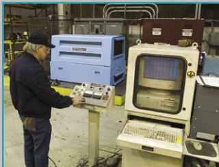
Load testing to 1,500 HP and 13.2 kV / 500 VDC
