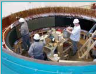
On-site hydro generator rewind
