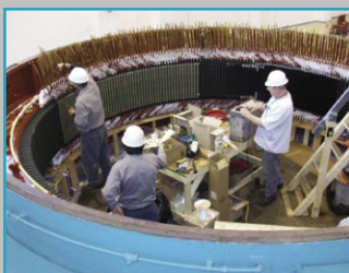
On-site hydro generator rewind
