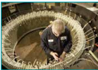
In-shop motor and generator repair
