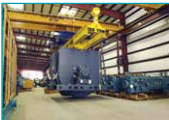
Critical equipment storage
