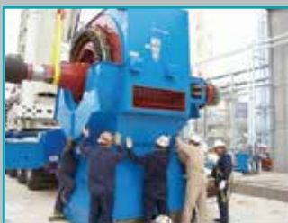
Extensive On-Site Field Services
