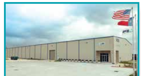
New, clean, temperature- and humidity-controlled 60,000 sq. ft. warehouse
