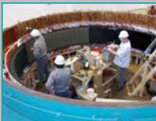
On-site hydro generator rewind
