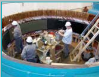
On-site hydro generator rewinds
