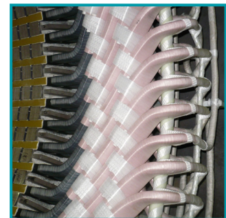
Reliable "Crossover" connections with extensive blocking, bracing & lashing
