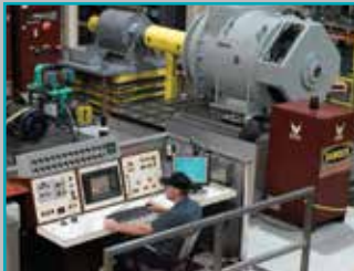
Load testing to 1,250 HP and 6,900 VAC / 750 VDC
