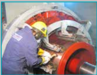
Dedicated Field Service Technicians
