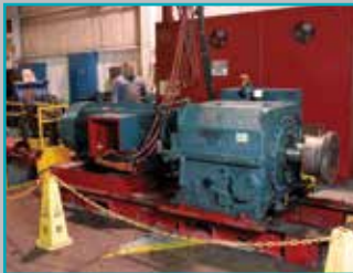
Load testing to 1,250 HP and 13,800 VAC / 750 VDC
