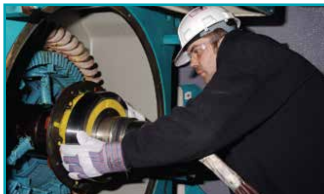
Bearing changeout on an ABB 1.5 MW generator
