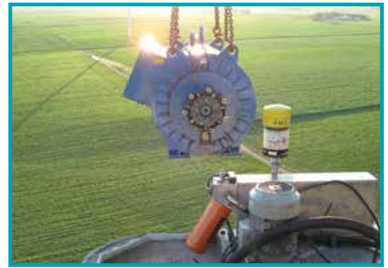
IPS technicians are trained and experienced in generator removal and replacement
