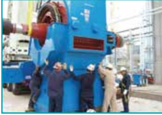
Extensive on-site field services
