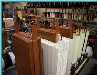
Transformer and Reactor repair
