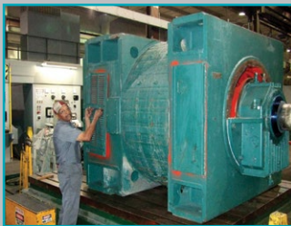
Run testing to 4,160 VAC / 700 VDC
