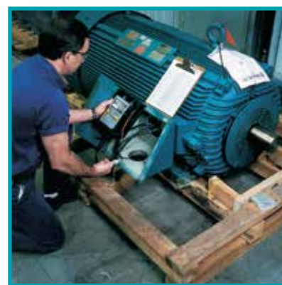
Coils are Meggered quarterly (or to customer specification)
