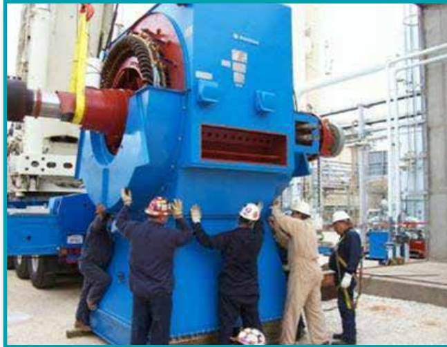
Commissioning of a 21,000 HP main air compressor motor.
