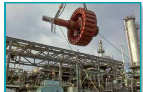
Installation of 7,000 HP synchronous rotor.
