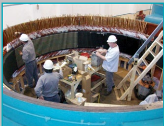
On-site hydro generator rewinds
