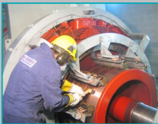
Dedicated Field Service Technicians
