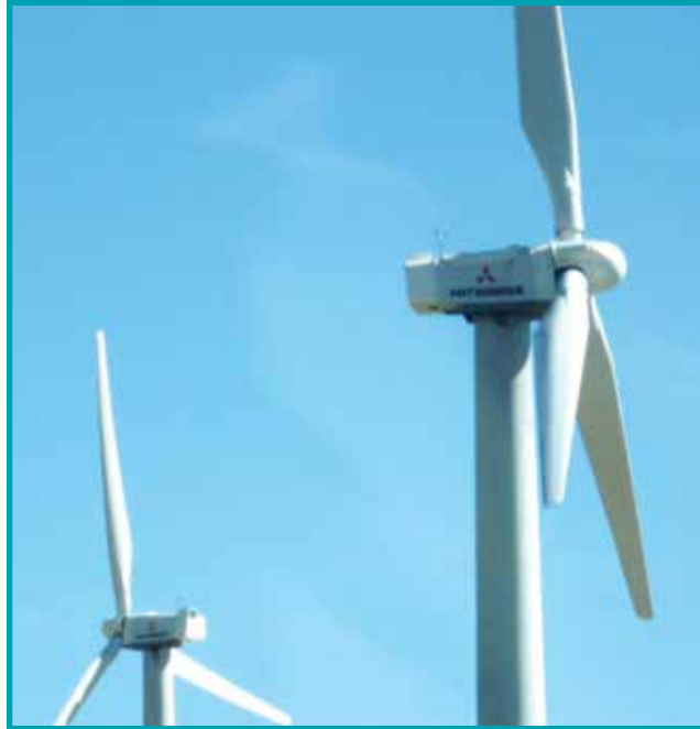
Our dedicated up-tower and in-shop technicians service Mitsubishi turbines coast to coast
