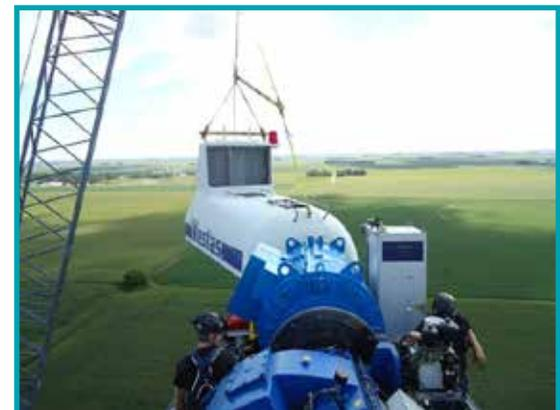
*IPS field service team installs replacement generator after removing failed unit*
