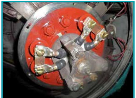
*IPS field service technicians have the equipment to test and repair rotor leads up-tower*
