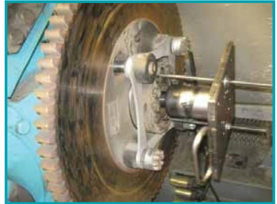
*IPS removes the generator brake up-tower to access the seals that cause hub slip ring issues*
