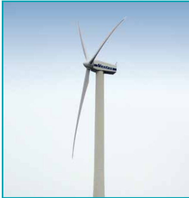
Our dedicated up-tower and in-shop technicians service Vestas turbines coast to coast
